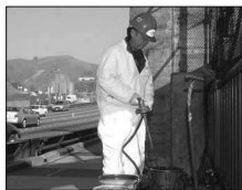
This worker is mixing an oil-based primer before painting the Golden Gate Bridge.
